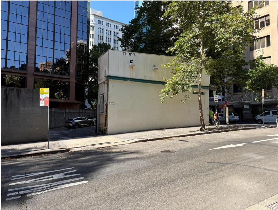
Figure 3: Site when viewed from the north side of Wynyard Street (south end of Wynyard Park)
